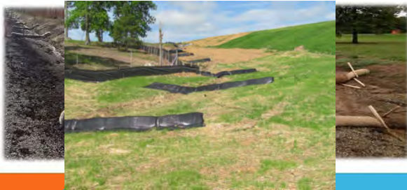
Alternate Ditch Checks
