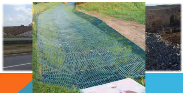
Channel and Slope Armoring
