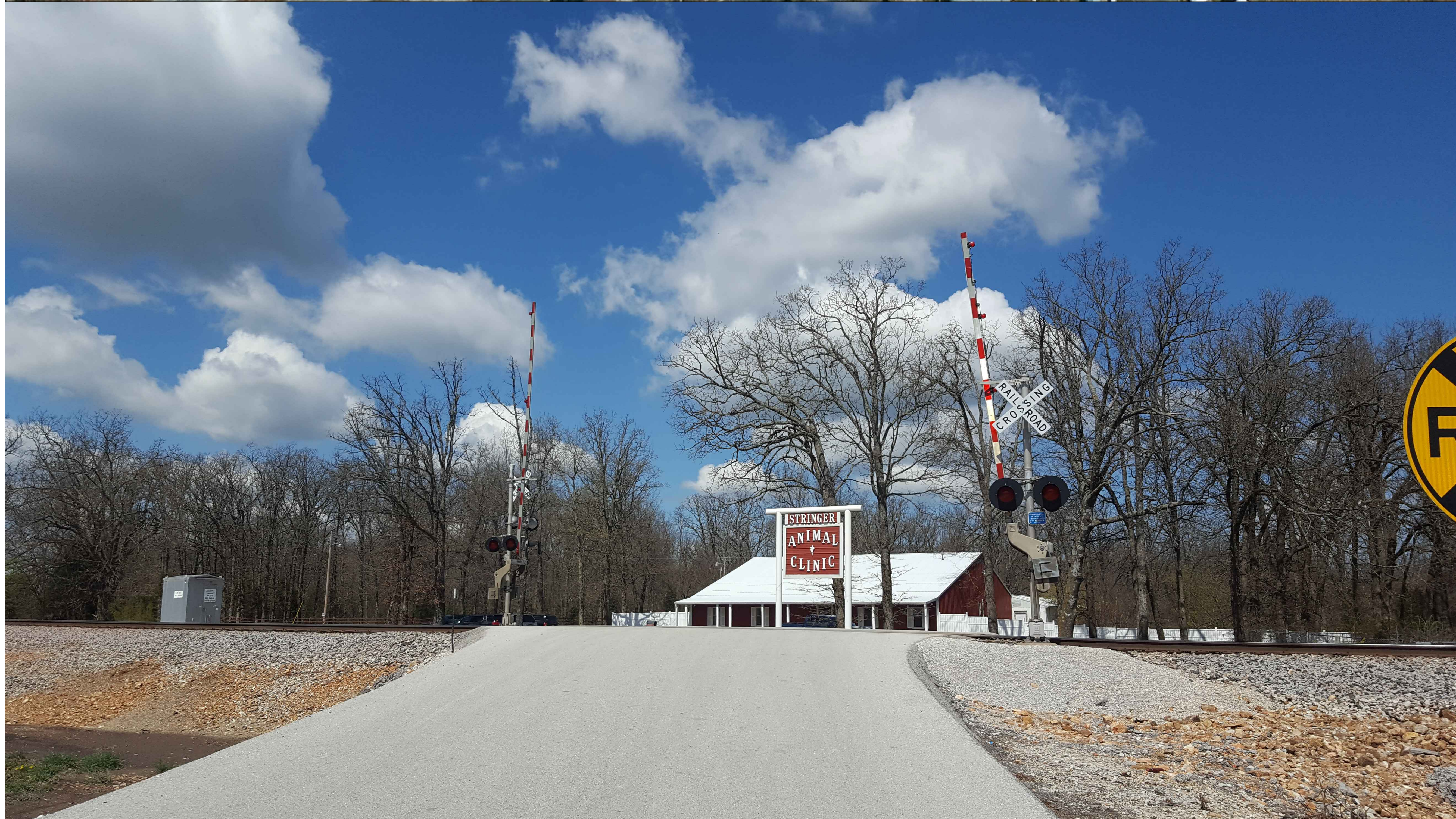
MoDOT - BNSF RAILROAD (CHEROKEE SUB-DIVISION FROM M.P. 248 TO M.P. 268) AT-GRADE RAILROAD INCIDENT SUMMARY
