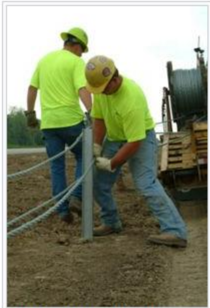
Installing low-tension guard cable
