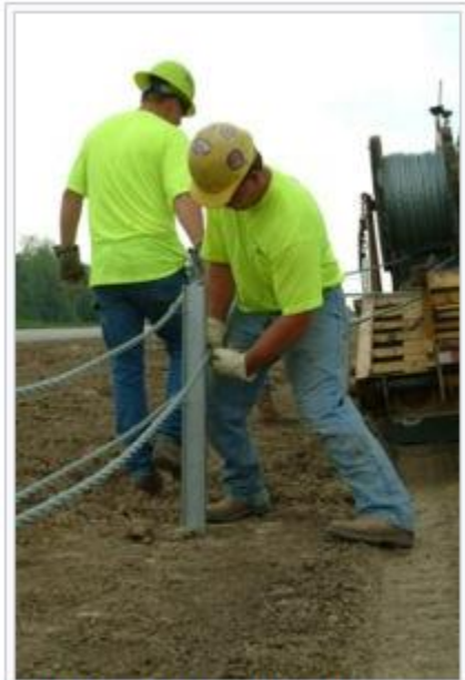
Installing low-tension guard cable
