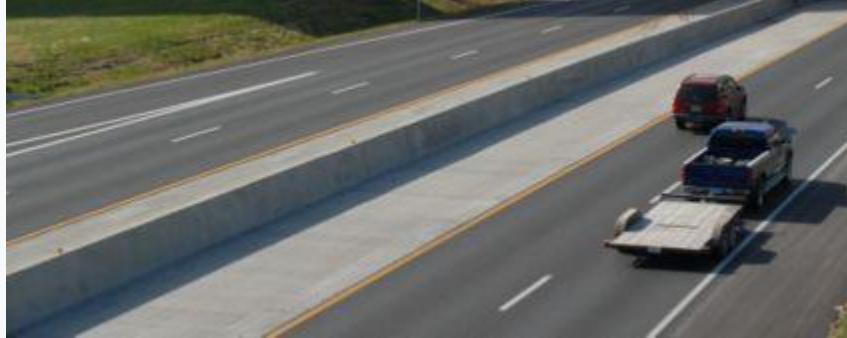
Type C Permanent Concrete Traffic Barrier
