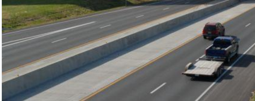
Type C Permanent Concrete Traffic Barrier
