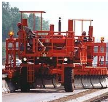
Moving the temporary concrete traffic barrier
