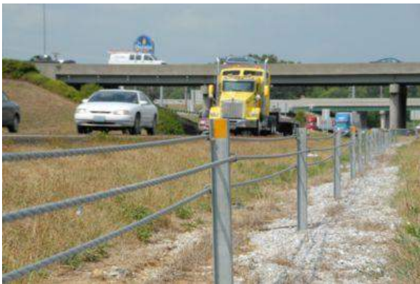
Low-tension Guard Cable
