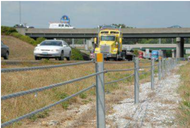
Low-tension Guard Cable
