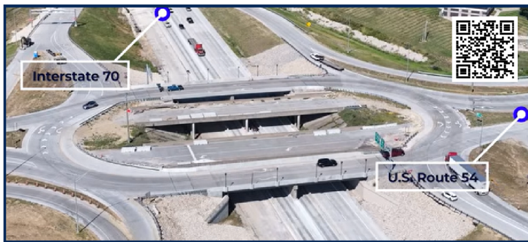
The new roundabout interchange at I-70 and U.S. Route 54 in Kingdom City.
