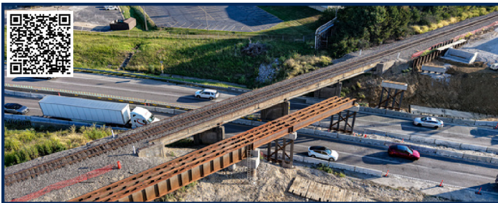
Girders have been set on temporary rail road bridge over I-70 in Wentzville.
