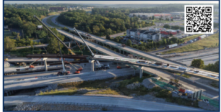
Steel bridge girders have been set on the new direct connection fly over ramp at I-70 and U.S. Route 63 in Columbia.
