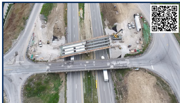
Construction is underway on the new Route D bridge over I-70 in Bates City.
