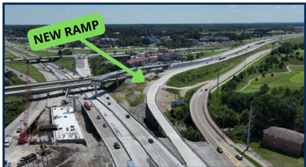
The new direct connection ramps provides access from eastbound I-70 to southbound U.S. 63 in Columbia.
