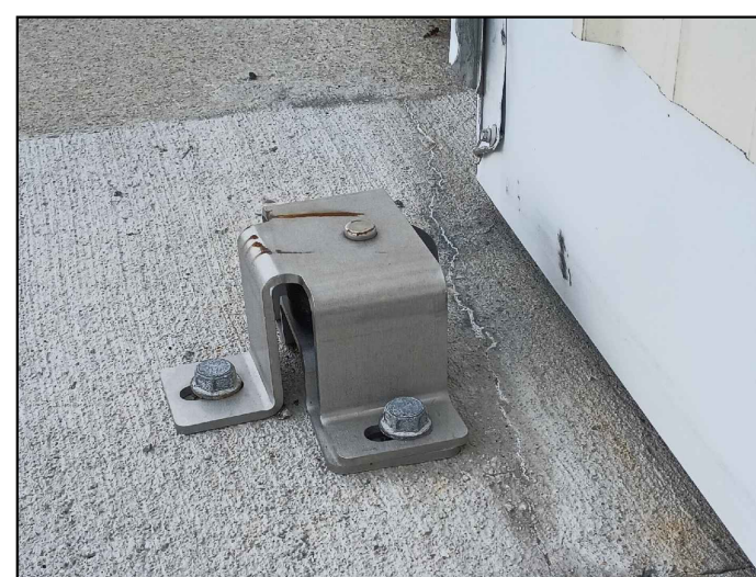
Existing Hangar Door Stop in Concrete Hangar Ramp
