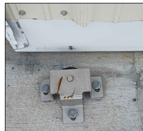
Existing Hangar Door Stop in Concrete Hangar Ramp
