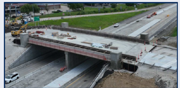
Construction of the new St. Charles Road bridge over I-70 is ahead of schedule.
