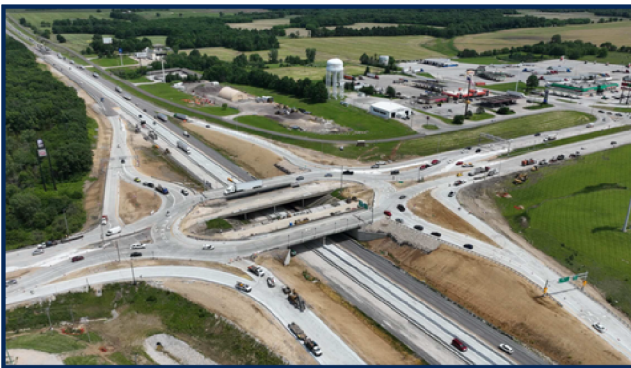
New I-70 and U.S. Route 54 interchange opens in Kingdom City.
