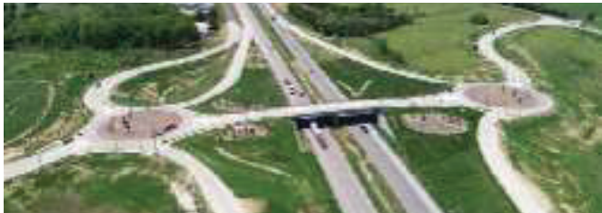
I-70 & Route MM Interchange – Warrenton, MO
