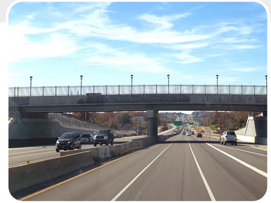
Project: I-270 North Design/Build Bonus Bridge
