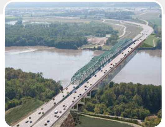
Project: I-64 Daniel Boone Bridge over Missouri River
