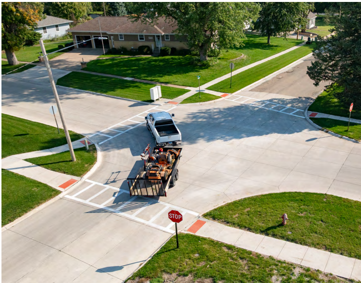
Street Improvements, Arlington, NE
