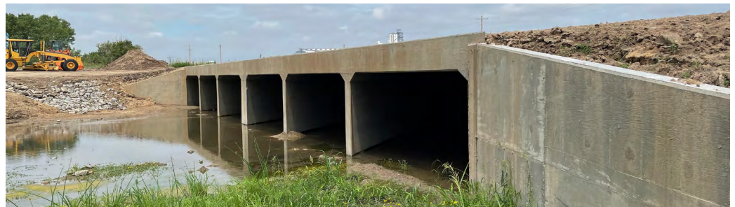
Mine Road Culvert, Hutchinson, KS ▶
