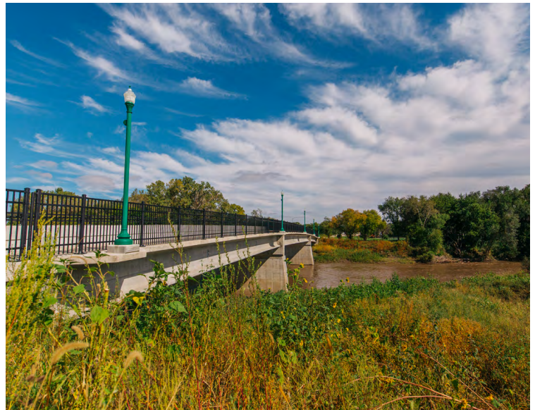
Silver Street Bridge Replacement over Salt Creek, NDOT LPA, Ashland, NE
