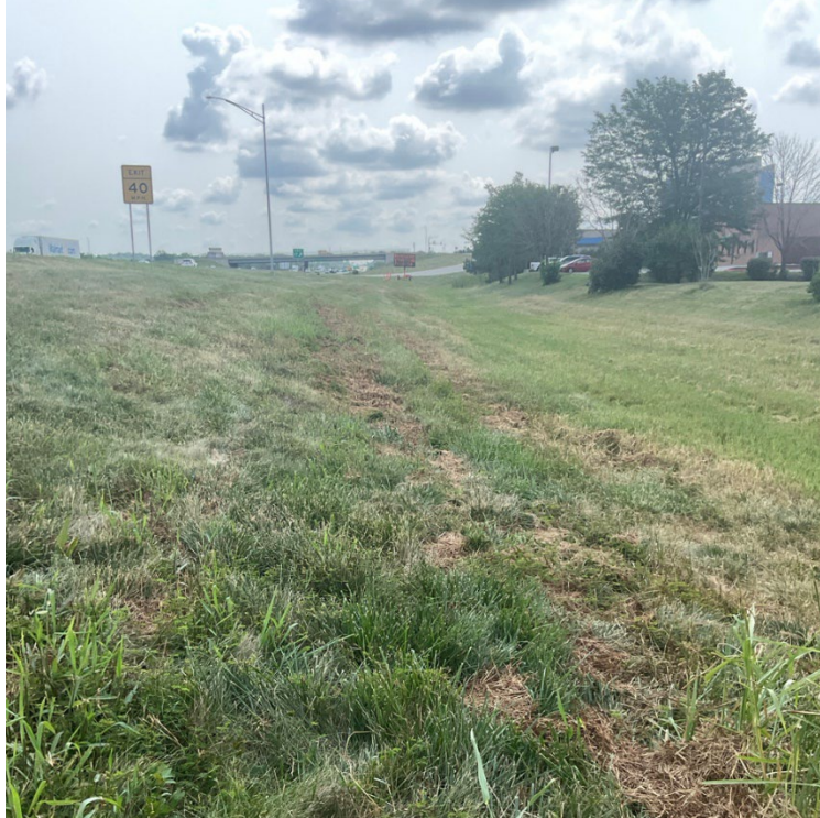
Photo 3: Overview of grass area near wetland area W10, facing east. Area designed for water to flow away from interstate (I-70) and parking lots, allowing to pool around the W10 location.
