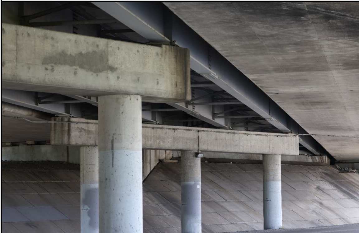
Photo 12: I-70 bridge overview in the central portion of the Project Area.
