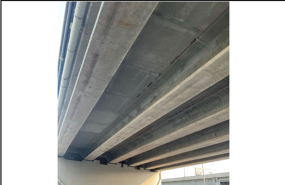
Photo 11: I-70 bridge overview in the western portion of the Project Area.
