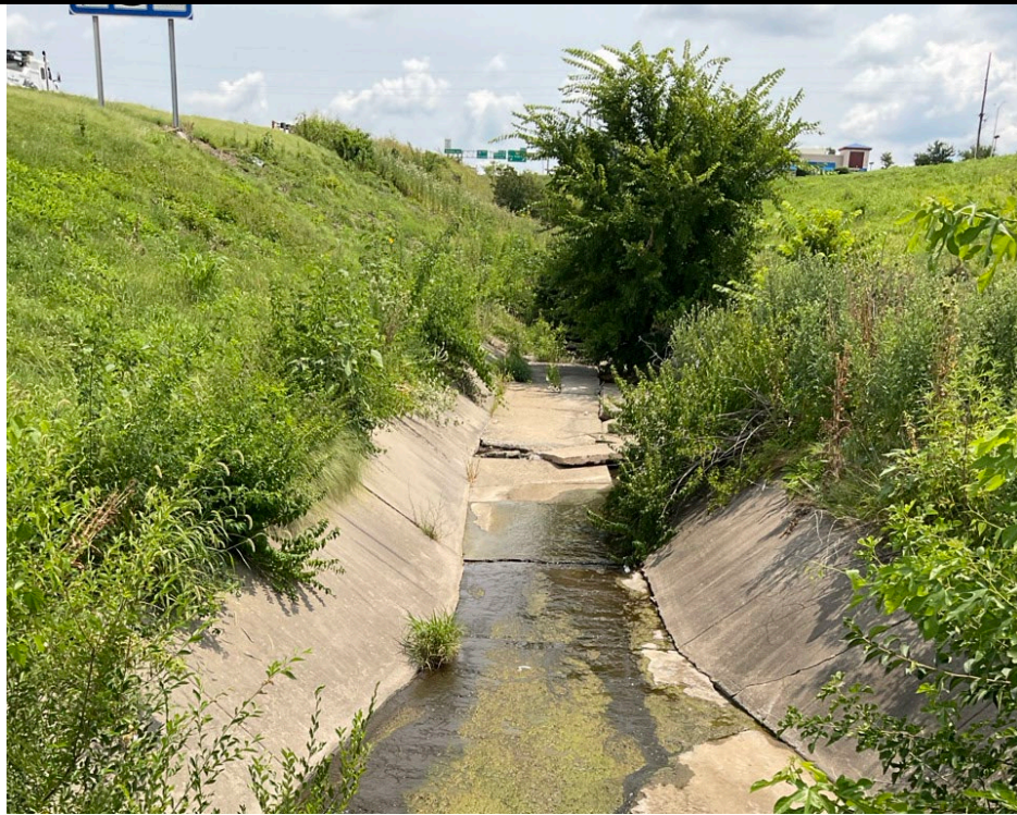
Photo 9: Culvert located along I-70.
