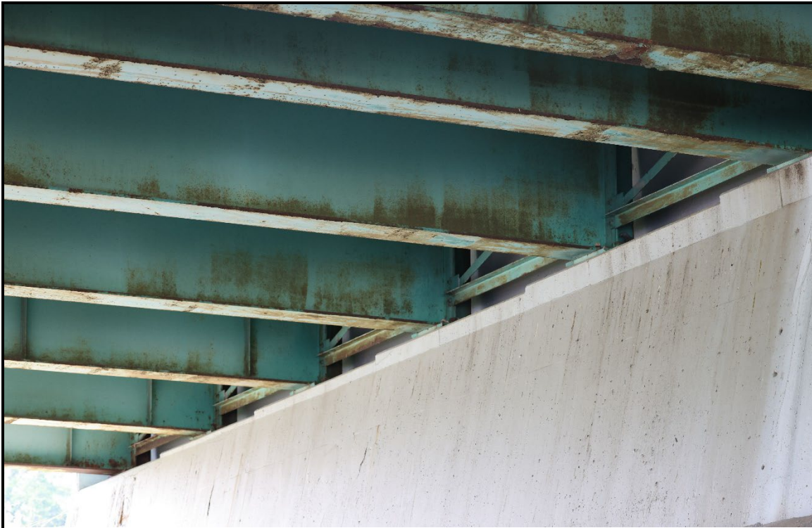
Photo 13: I-70 bridge overview in the eastern portion of the Project Area.
