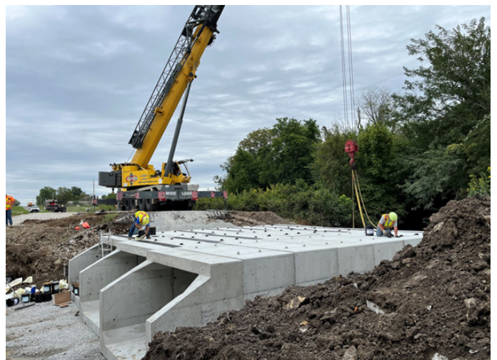
Crews install a box culvert in Polk County.
