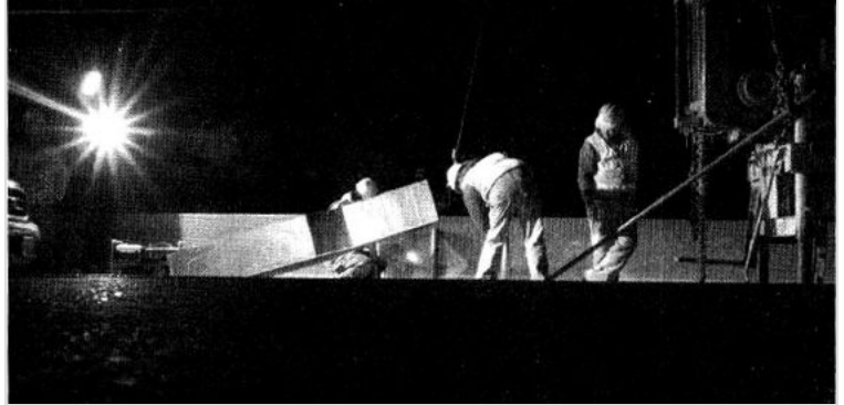
Crew takes a soil sample on an interstate to determine soil conditions and how much rock is beneath the surface.
