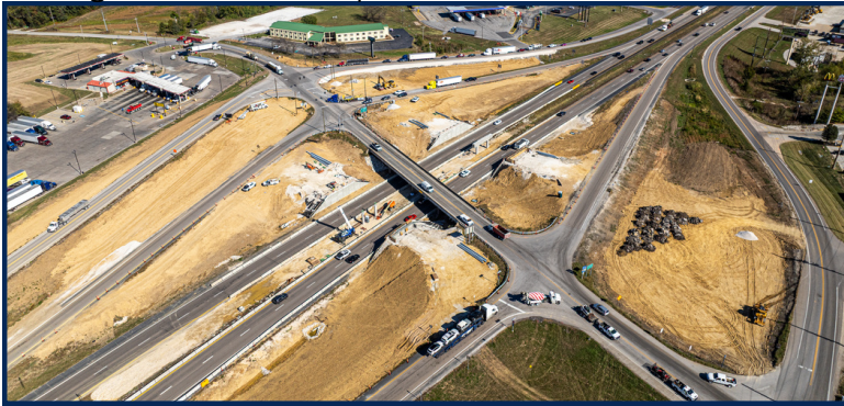
Bridge work is ongoing at the Route T/W interchange in Foristell.
