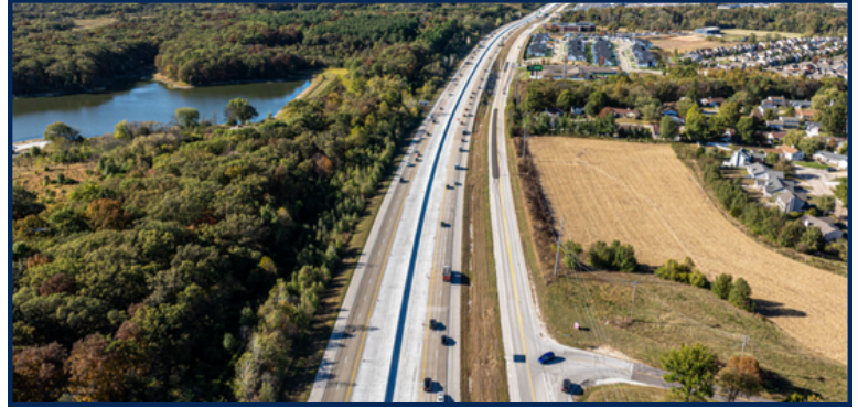
Crews continue to make paving progress along I-64 between I-70 and Route K.
