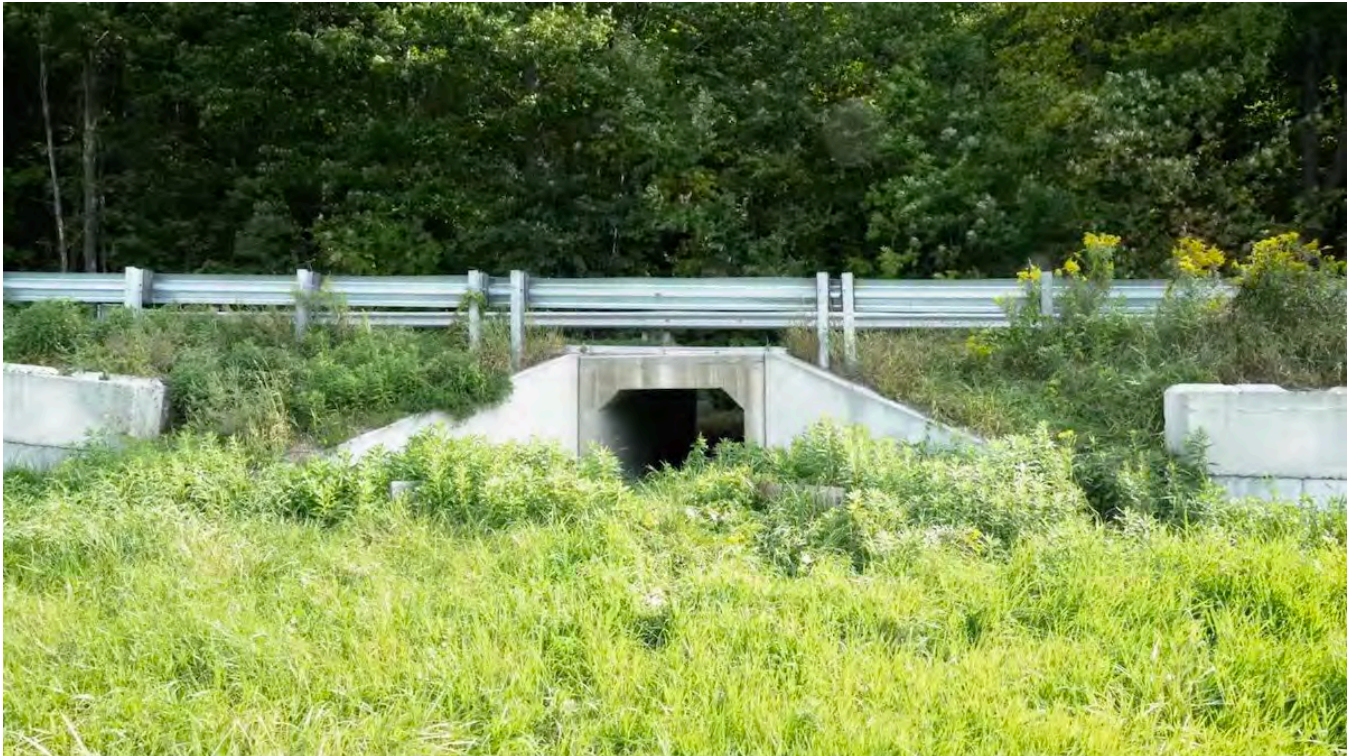
A wildlife underpass tunnel installed under a road in Monkton, Vermont to help pass small- and medium-sized animal species, and specifically to help amphibians. Credit: Vermont Agency of Transportation.
