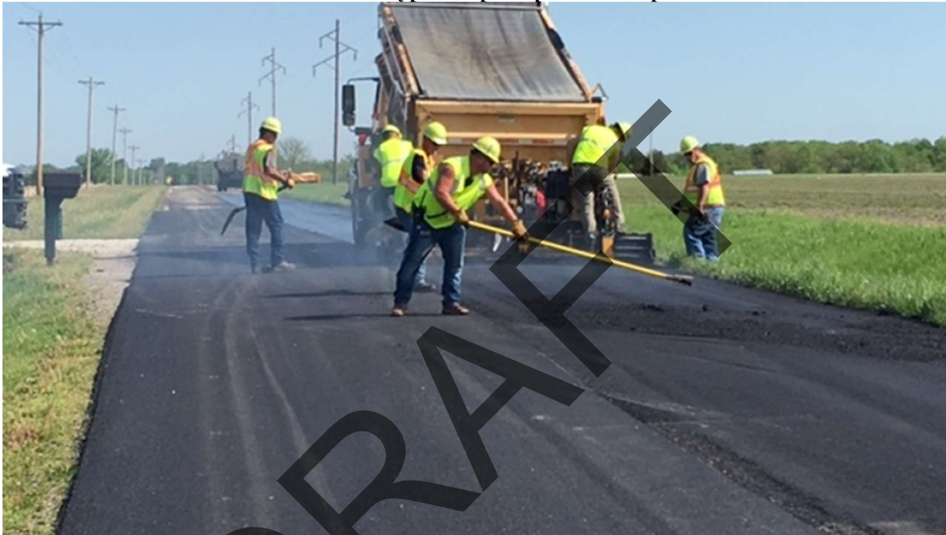
Typical asphalt pavement repair
