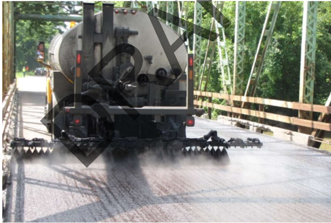
Typical bridge sealing
