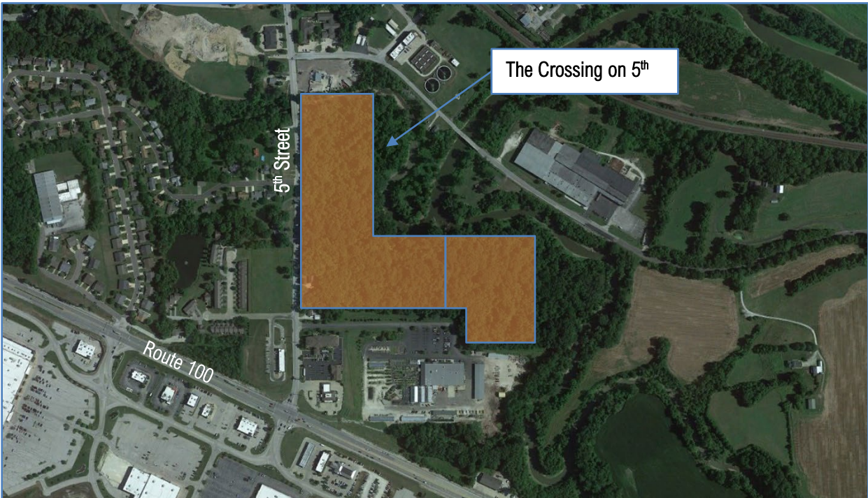
Figure 4: The Crossing on 5 th Development Area (under Construction)
