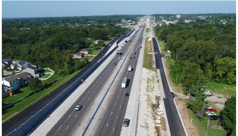
Currently, the Westbound I-270 to Northbound 367 ramp is closed. New asphalt is being installed on I-270 eastbound and westbound, along with the outer roads, cross streets, and shared use paths. Striping activities will be follow this operation around until the work is complete.
