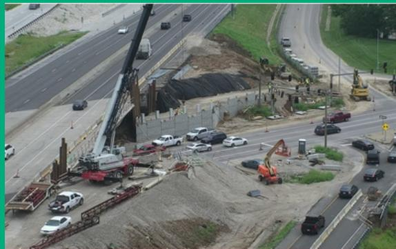
Crews prepare to drive pile for the new bridge at New Halls Ferry on August 10.
