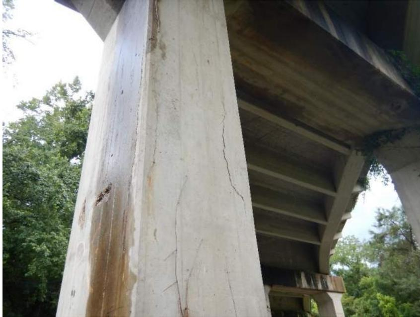
Deterioration of Intermediate Bent Columns
