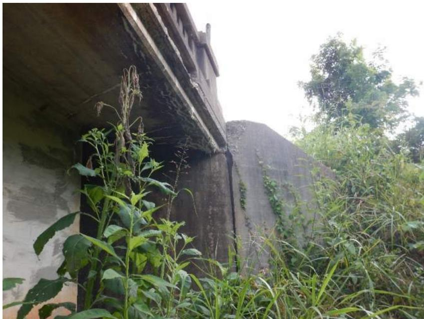
Typical Spalling at Abutment
