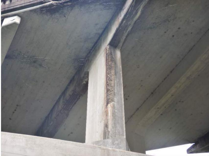
Typical Deterioration on Spandrel Columns
