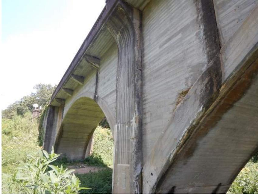
Spalling on Pier Surfaces
