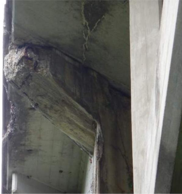
Typical Deterioration of Brackets
