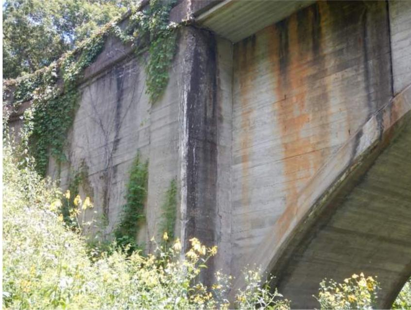
Cracking and Delamination at Abutments
