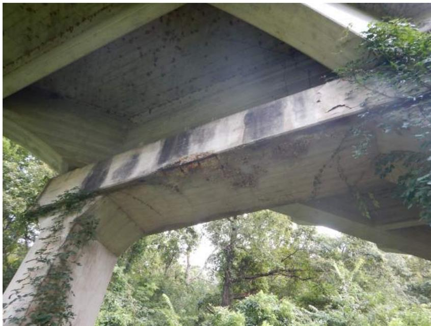
Deterioration of Intermediate Bent Cap Beams
