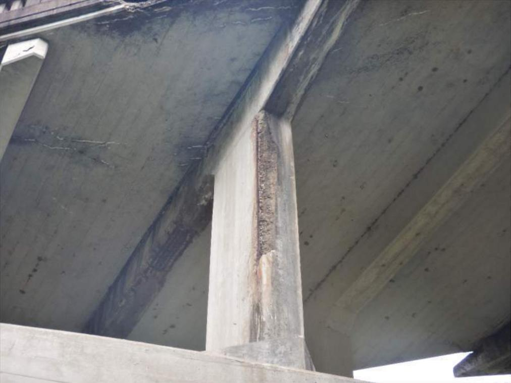
Pic. 010: Vertical cracking in column, Bent 3 shown
