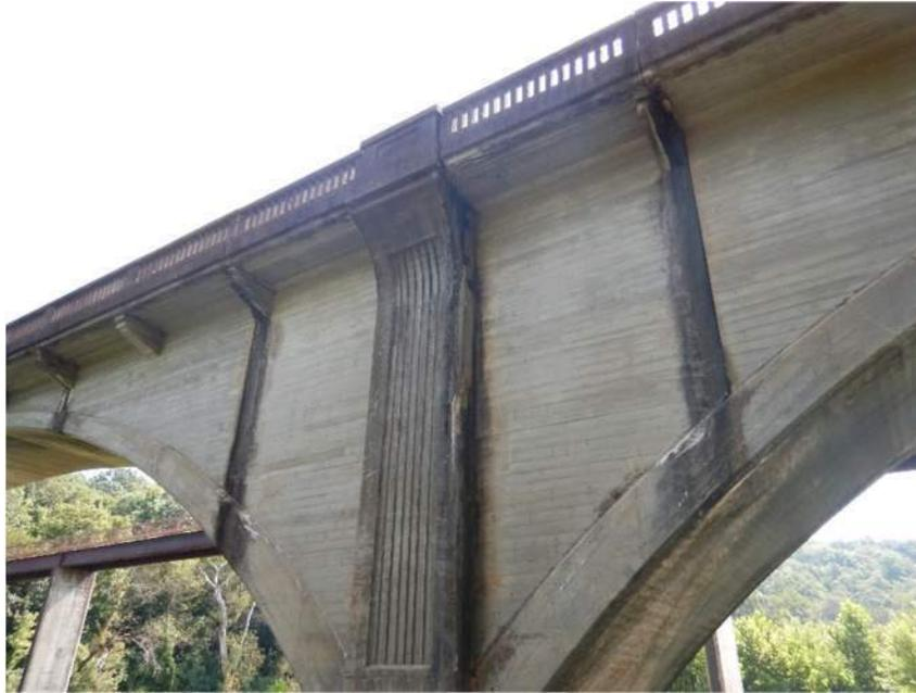
Leakage from Sidewall Joints
