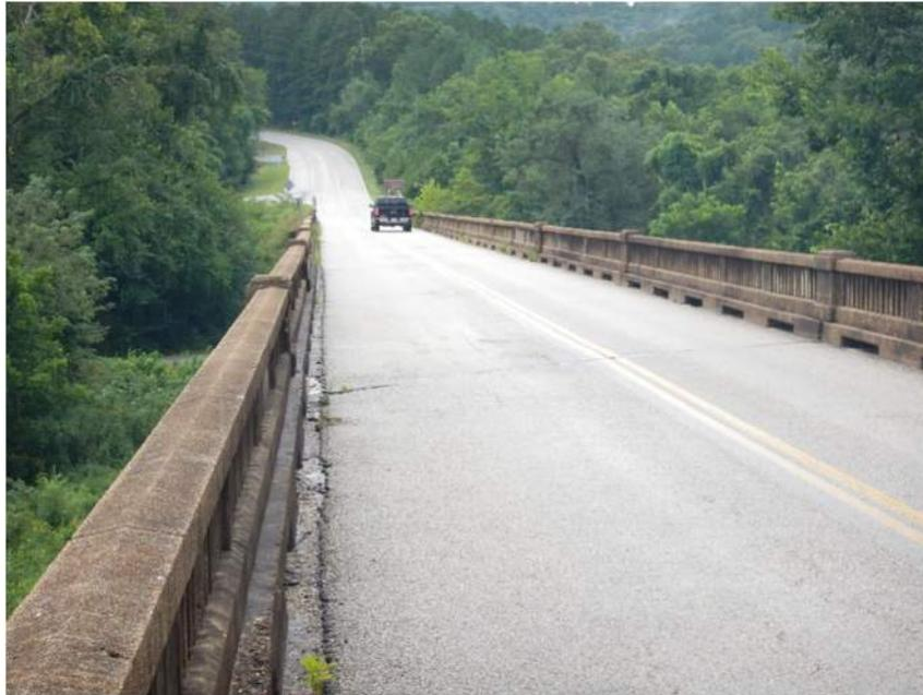
Collision Damage to the Railing
