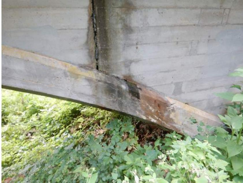
Spalling and Staining on Arch Ring
