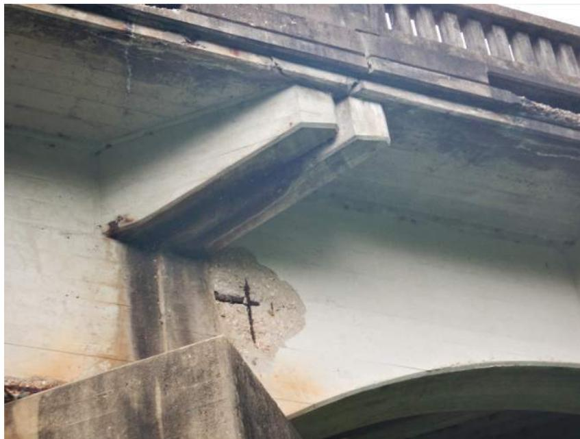
Typical Delamination on Girders
