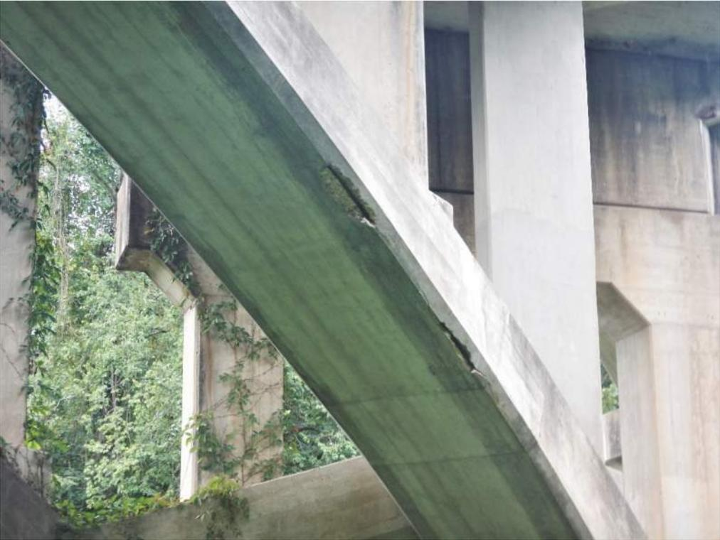
Pic. 009: Typical deterioration of spandrel column
