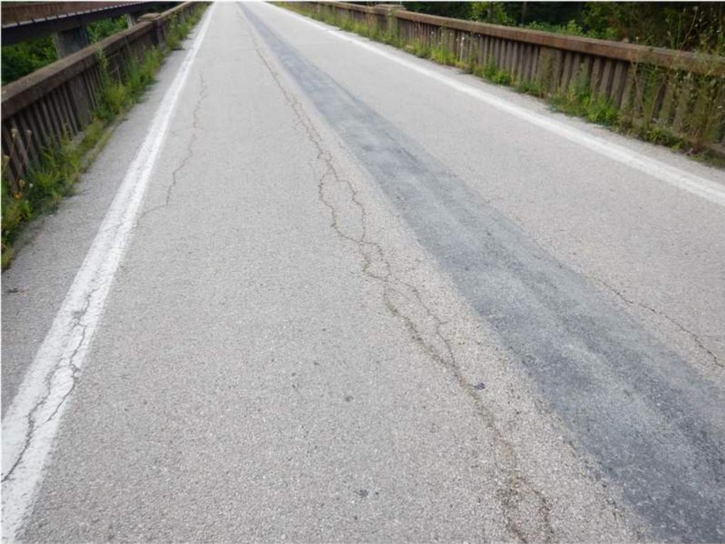
Pic. 002: Typical leakage from sidewall joints
