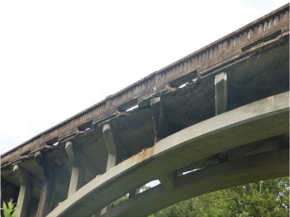
Pic. 003: Bridge barrier rail with misalignment
