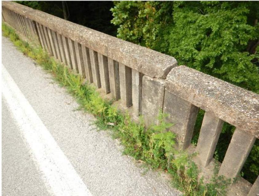
Collision Damage to the Railing
