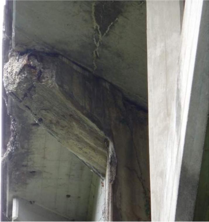
Pic. 006: Typical deterioration of spandrel capbeams
