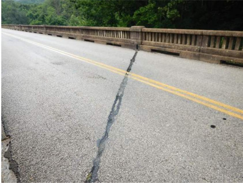
Typical Slab Expansion Joint
