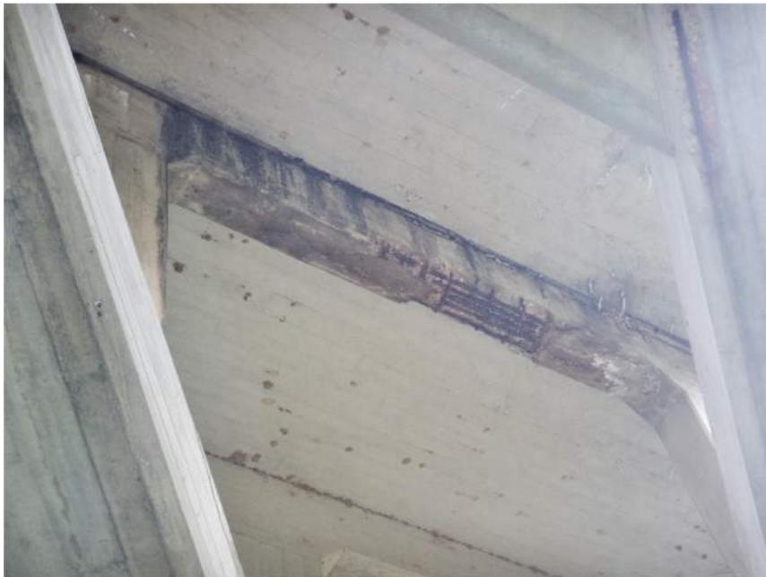
Typical Deterioration on Spandrel Capbeams
