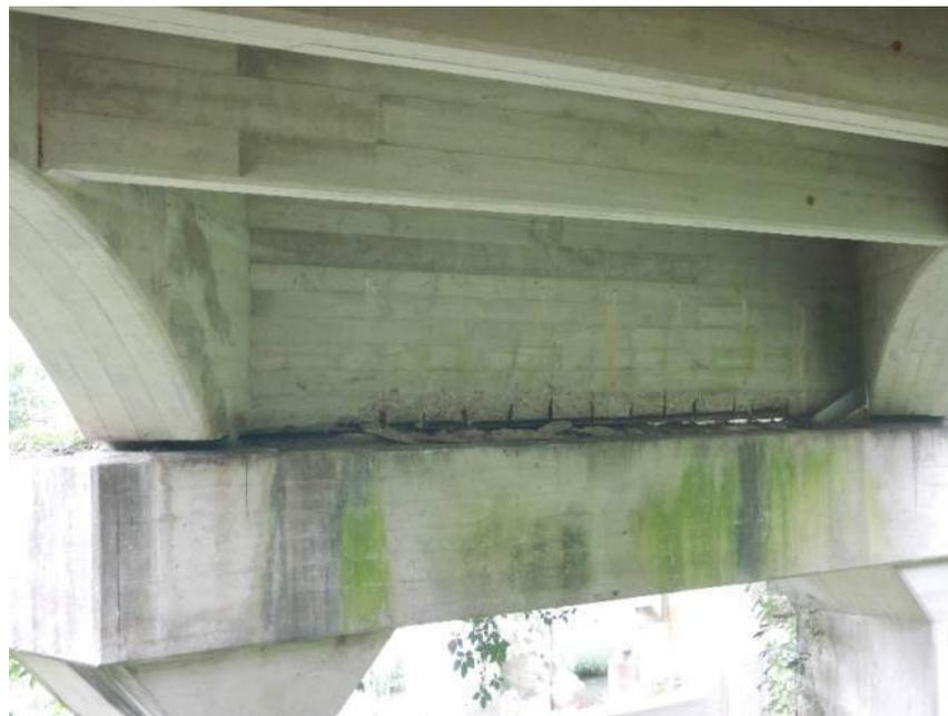
Deterioration of Floorbeams at Intermediate Bents
