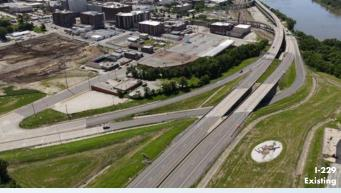
In this alternative the double-decker bridge is removed and replaced with a new four-lane arterial road constructed at-grade (elevated as necessary for compliance with floodplain and stormwater requirements) in generally the same location as the existing double-decker bridge between the railroad tracks and the Missouri River. This alternative would require de-designation of I-229 as interstate.
