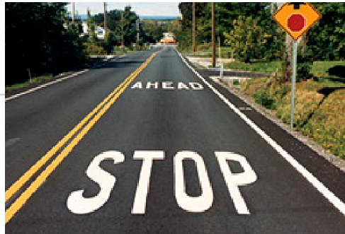
Figure 12: “STOP AHEAD” markings and sign
