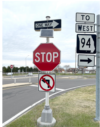
Figure 13: LED stop sign with a solar charger
