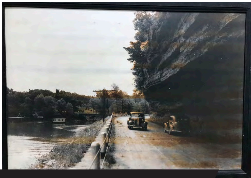
Early cable barrier separating traffic from embankment to the Elk River, Noel, Missouri.
