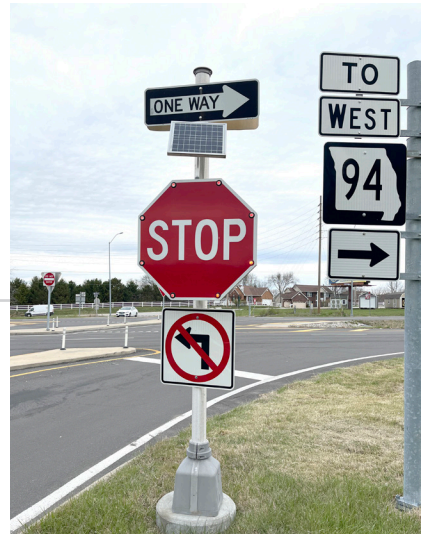
Figure 13: LED stop sign with a solar charger
