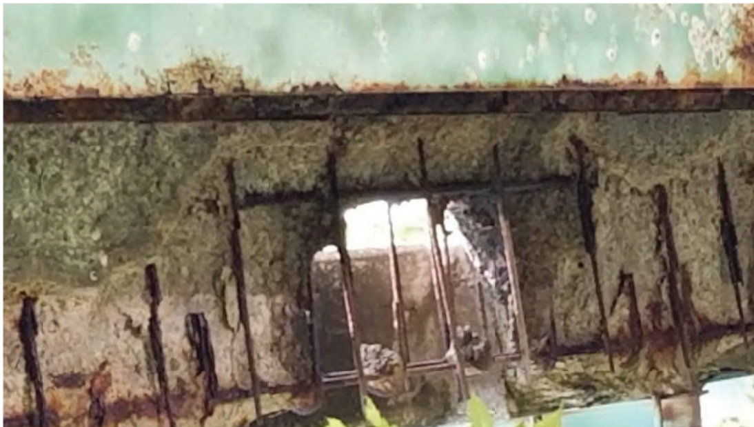
PHOTO 6 - DECK DETERIORATION (EAST OVERHANG, MIDDLE SPAN)
