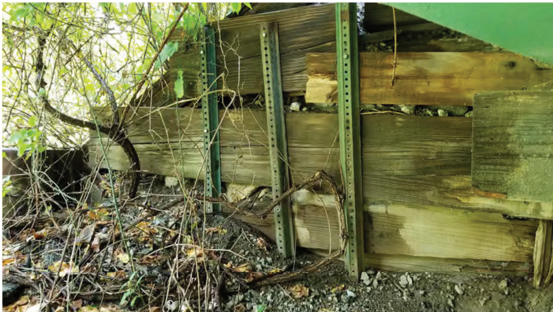
PHOTO 12 - WEATHERED AND MISSING TIMBER BACKING (NORTHWEST WINGWALL)
