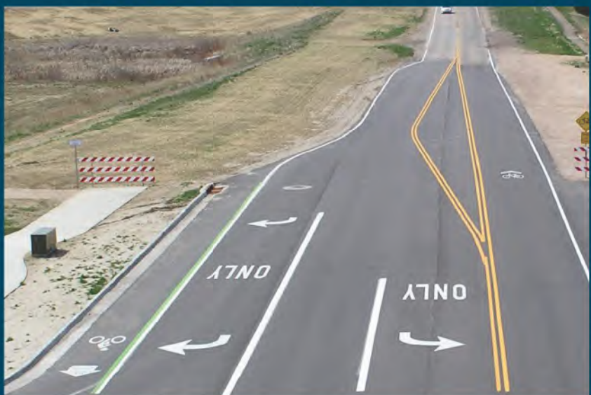
Left- and right-turn lanes on a two-lane road. Source: City of Greeley, CO
