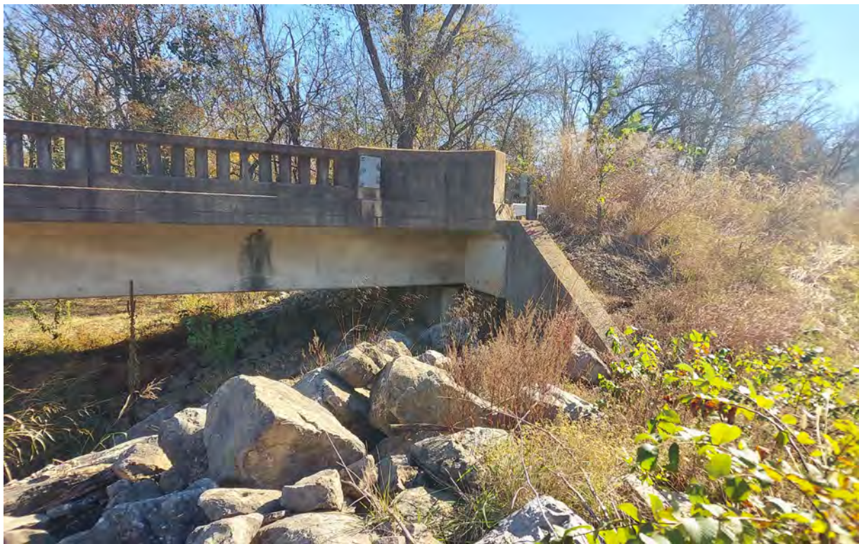
Photo 2. Southeast End Bent
