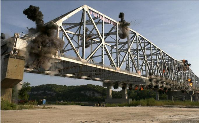
**Controlled blasts demolish the old I-70 Missouri River bridge at Rocheport.**
