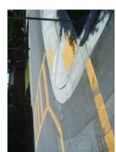
Diagonal Curb Ramps or corner type curb ramps are no longer preferred design types. A design that provides individual ramps for each crossing direction is recommended by the US Access Board.
