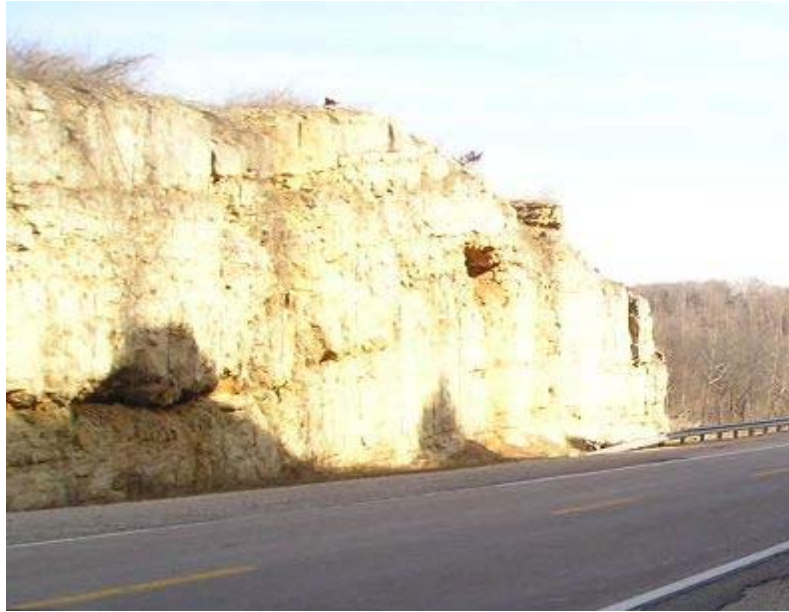
Existing rock cut along Route 63 at the Gasconade River Bridge shows solutioning activity, voids and clay filling.
