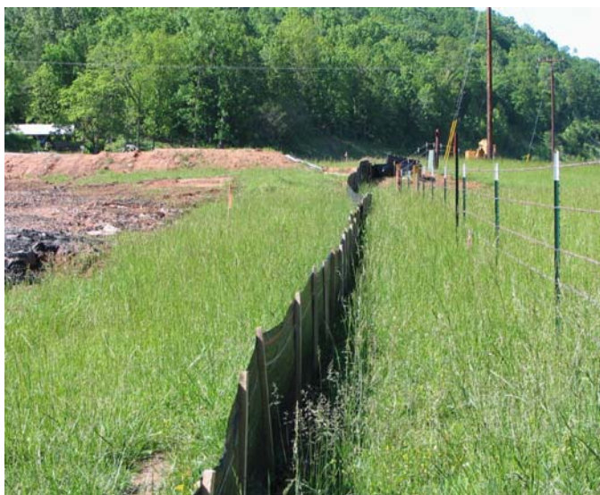
Silt fencing is most effective to control sheet erosion along the edge of the right of way where runoff from erodible fill could go onto adjacent property or into an adjacent stream.
