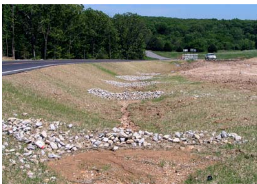
Some examples of temporary erosion control in ditches – silt fence and rock ditch checks are often used depending on the grade of the ditch.
