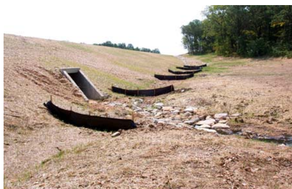
Some examples of temporary erosion control in ditches – silt fence and rock ditch checks are often used depending on the grade of the ditch.
