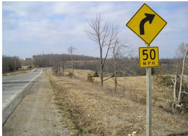
Typical section of Route 63, with four-foot gravel shoulders near Freeburn
