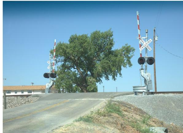
The cost to reprofile vertical grades is estimated to be \$50,000 per crossing at a conceptual level, though further study and detailed engineering analysis is required to refine costs for roadway re-profiling.
