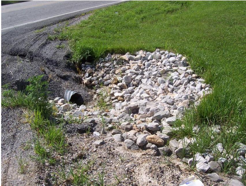
**Figure 6.13 Drainage improvements at the intersection of St. Charles Road and Route Z (Rossy et al., 2009).**
