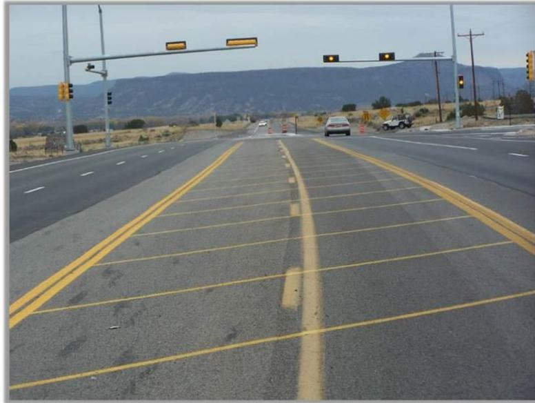
**Figure 6.6** Overlapping sets of pavement markings.
