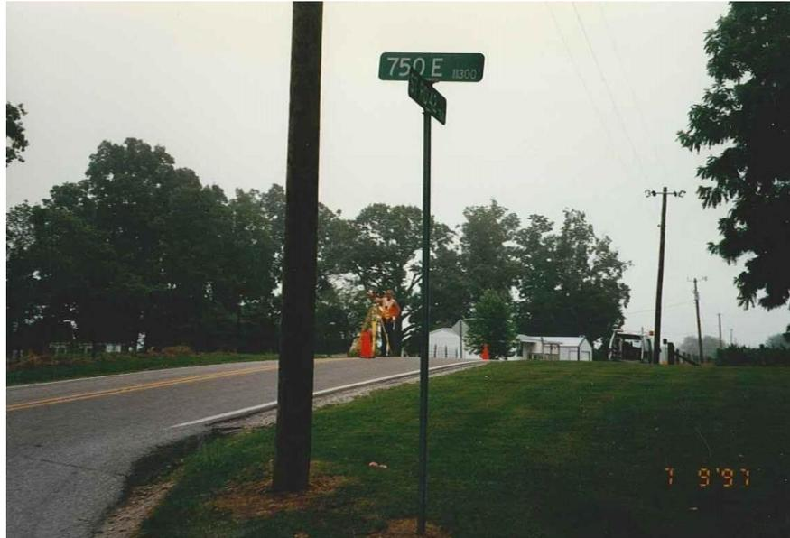
Figure 6.2 Intersection sight distance obstructed by hill.
