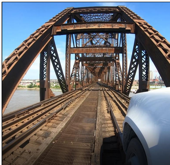
Figure 4 -- Typical Open Deck Layout with Rail Expansion Joint
