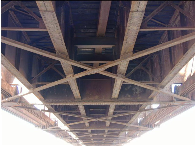
Figure 1 -- Typical Jack Stringer and Floor System Layout
