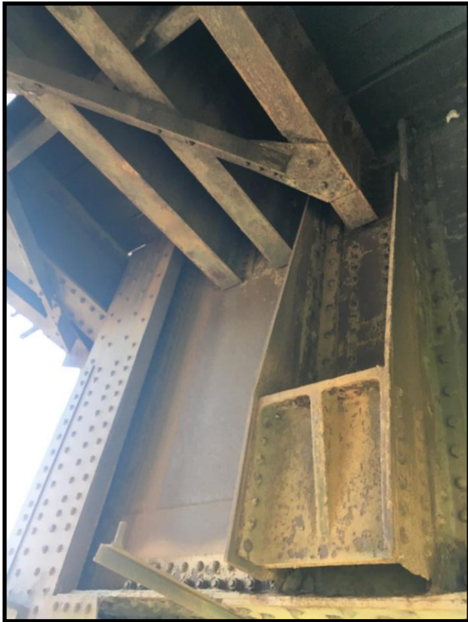
Figure 12 -- Modification to East Approach Bent E3 with North Approach Stringers shown
