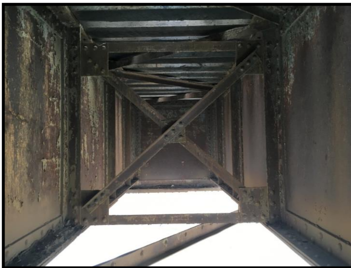
Figure 7 -- Interior of Typical Stringer Panel in Main Spans
