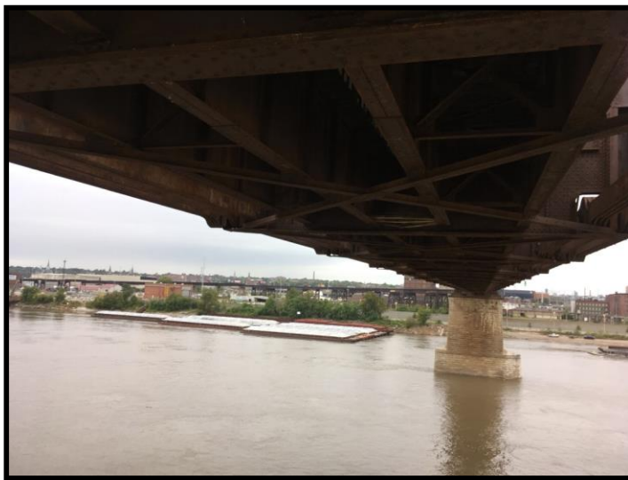
Figure 5 -- Main Span Floor System
