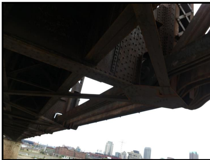
Figure 6 -- Main Span Floorbeam and Bottom Lateral Connection
