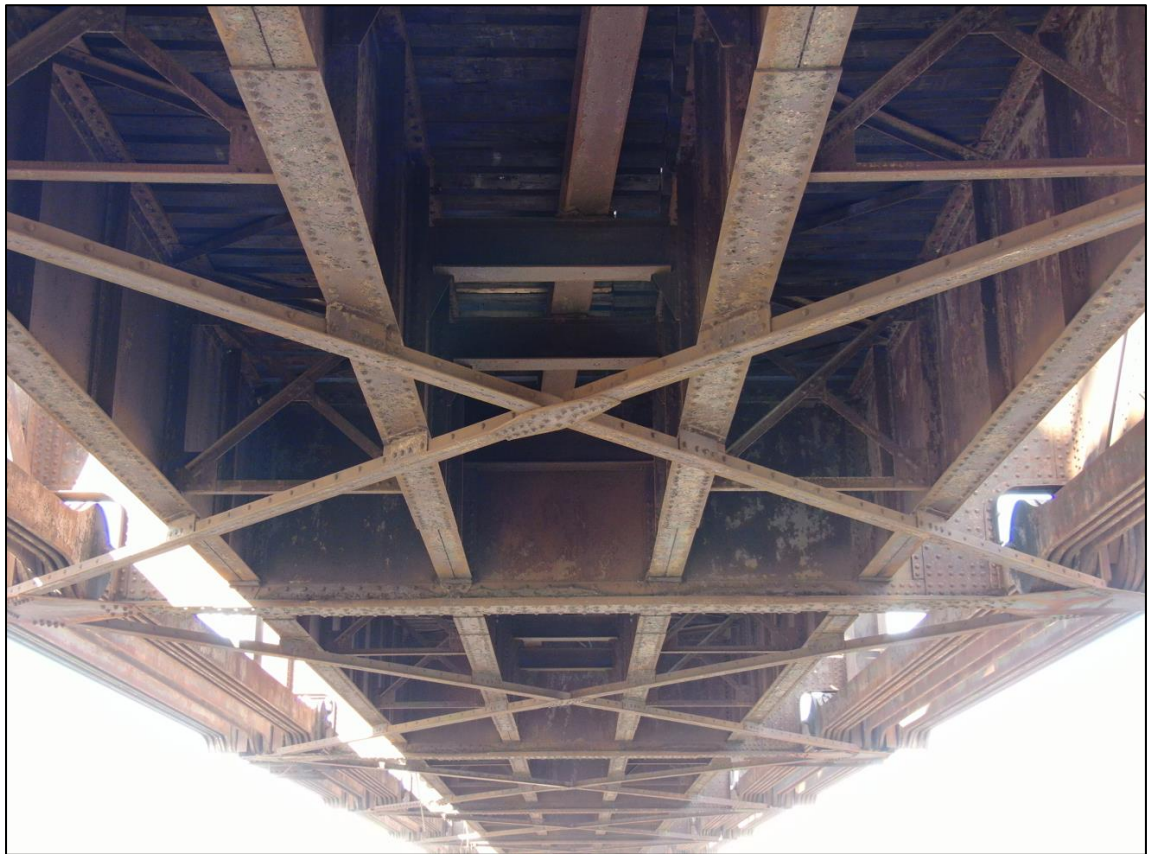
Figure 1 -- Typical Jack Stringer and Floor System Layout
