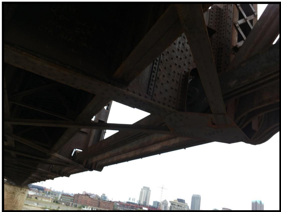
Figure 6 -- Main Span Floorbeam and Bottom Lateral Connection
