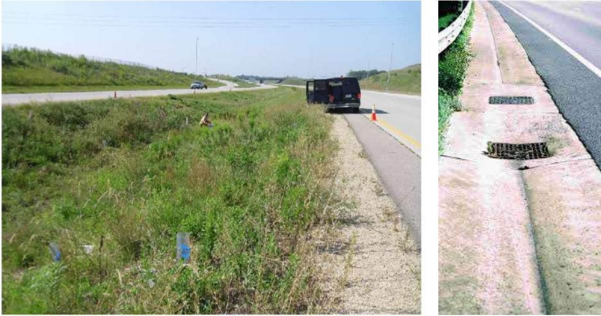
Figure 3-13. Photos of Typical Open and Closed Drainage Systems
