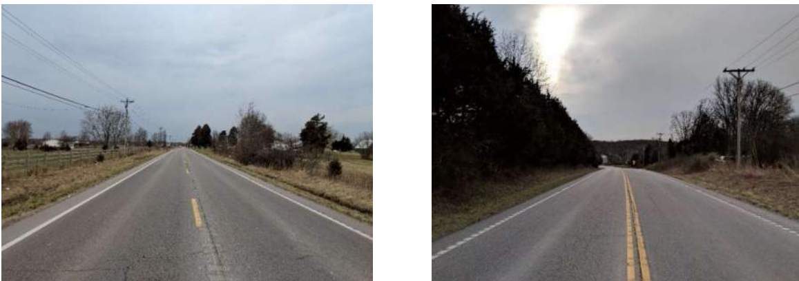
Figure 3-2. Typical Views along the Rural Portion of Route N
