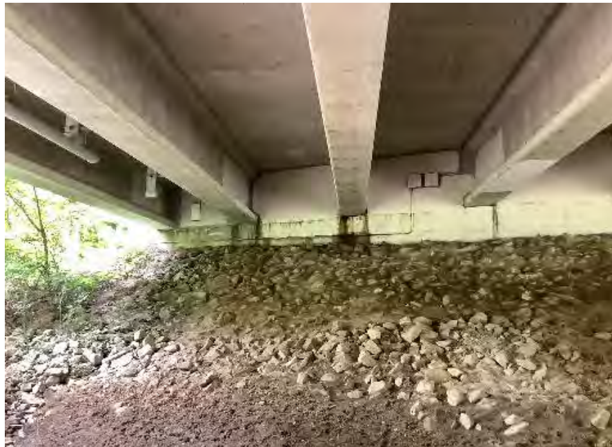
East abutment leaking
