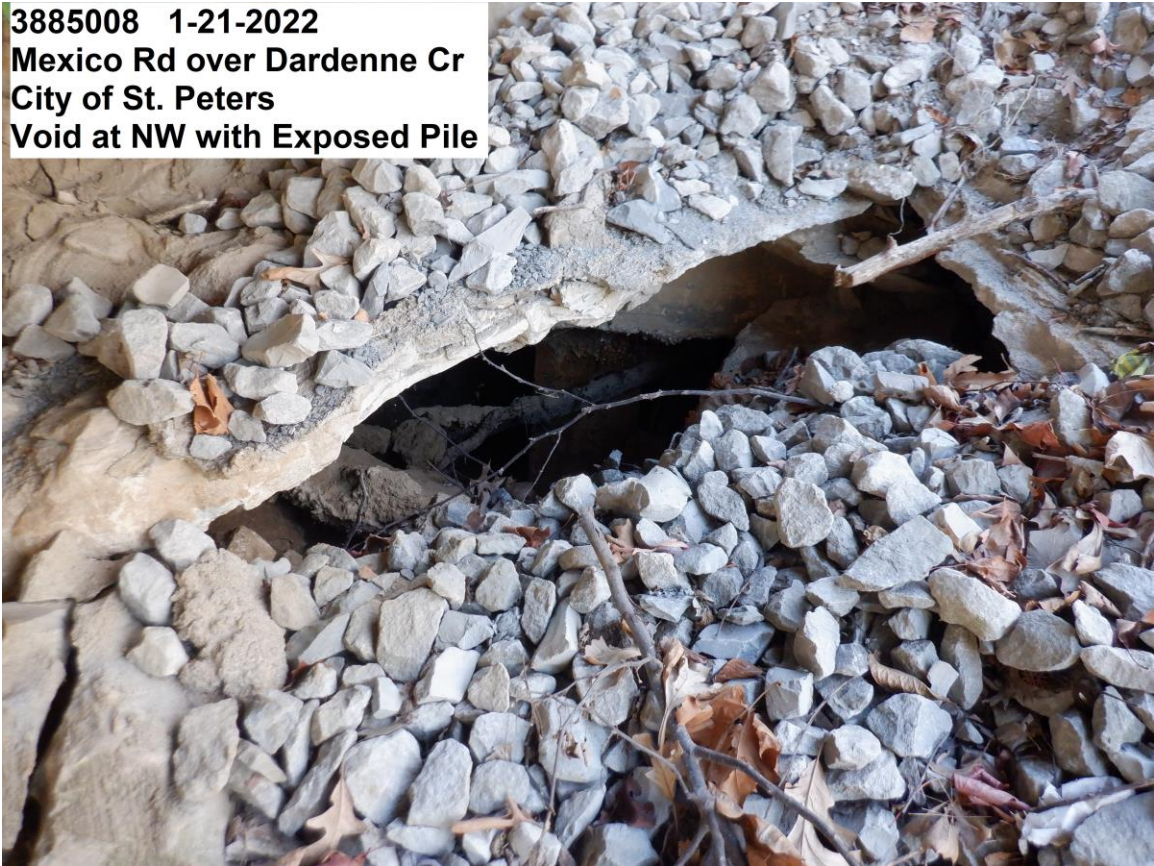
3885008 1-21-2022 Mexico Rd over Dardenne Cr City of St. Peters Void at NW Quad - Exposed Pile
