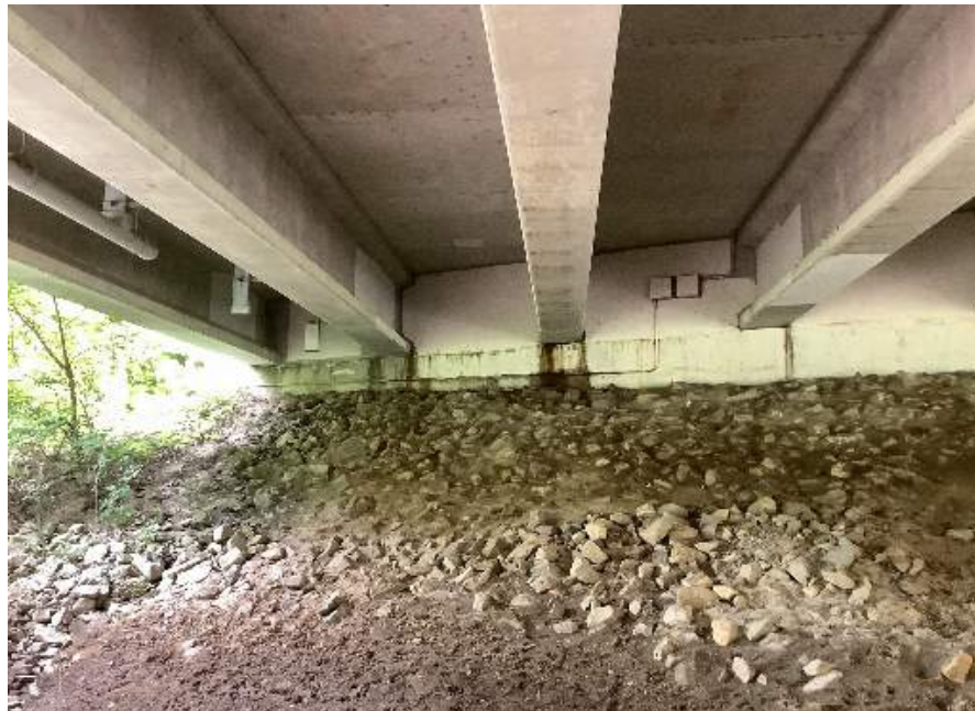
East abutment leaking
