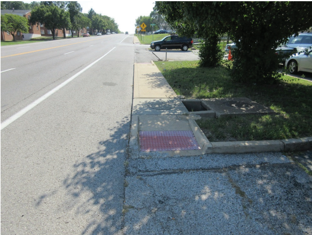
Figure 6: Southwark Lane to Ripa Avenue (looking South at Clyde Avenue)
