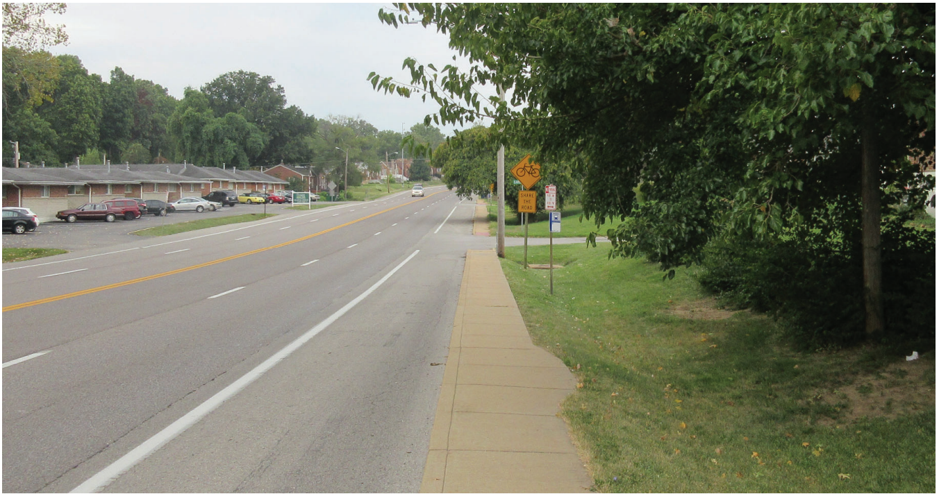
Figure 11: Metro Bus Stop Landing Pad (looking South at Southampton Drive)
