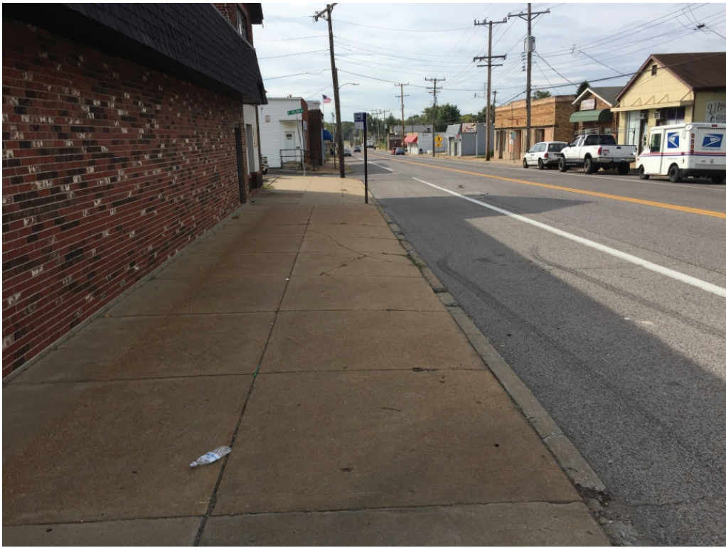
Figure 7: Ripa Avenue to Hoffmeister Avenue (looking South at Velma Avenue)
