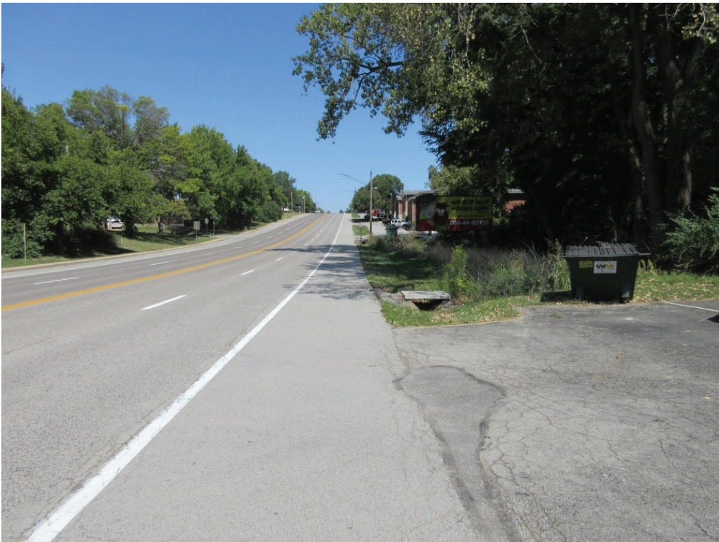
Figure 5: Southwark Lane to Ripa Avenue (looking North at Southwark Lane)
