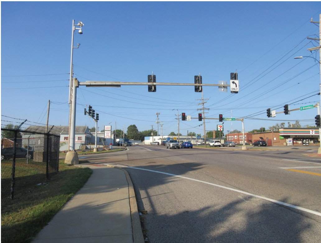
Figure 15: Route 231 at Hoffmeister Avenue (Southbound)
