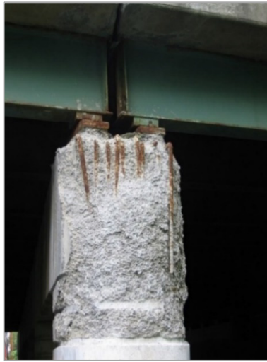
Figure 1. Photo. Reinforced concrete bridge substructure deterioration due to failed joint.
