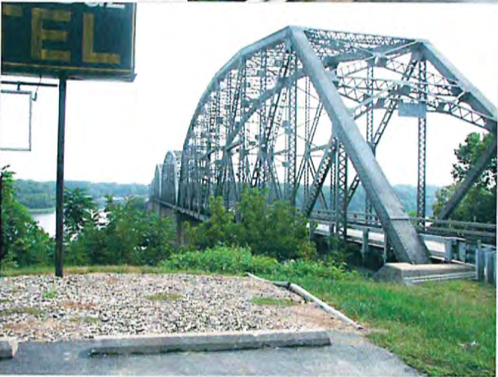
Bridge K0932, facing southeast
