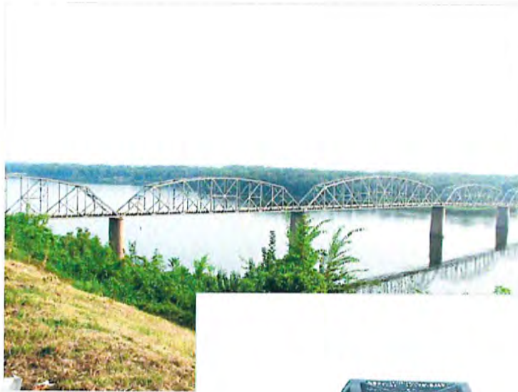
Bridge K0932, facing northeast
