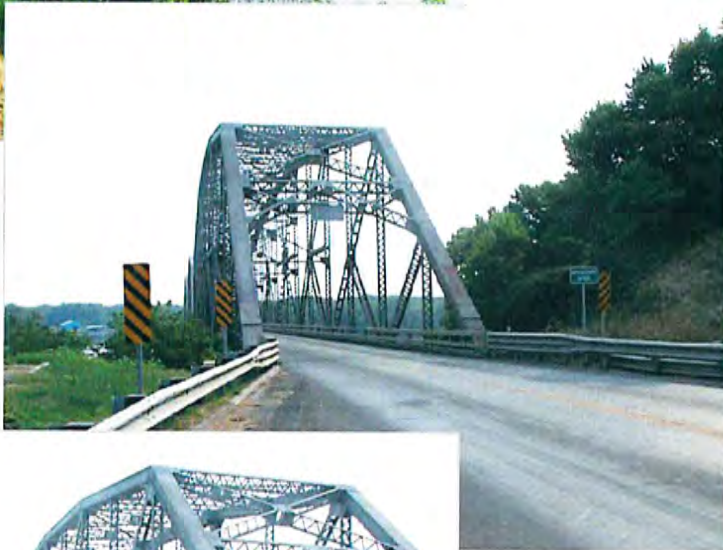
Bridge K0932, facing east
