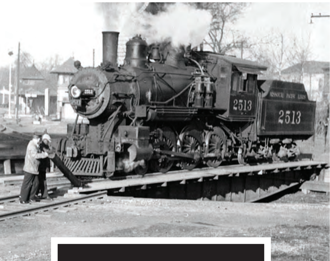
Kirkwood was the terminus for commuter trains operating between Union Station and Kirkwood. A 65-foot, hand-operated Armstrong turntable located near the present day Farmer's Market, allowed two men to turn around a locomotive for the trip back to Union Station. Photo taken on March 8, 1940. Photo source: Kirkwood Historical Society
