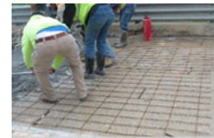
Wire mesh in the negative moment region
