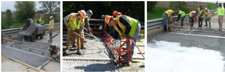
Figure Resource: UHPC overlay on Mud Creek Bridge deck, Iowa, 2017
