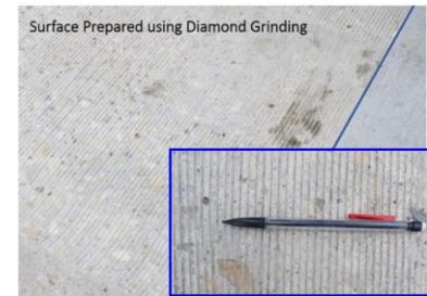
Scarification (UHPC overlay on Mud Creek Bridge deck, Iowa, 2017)
