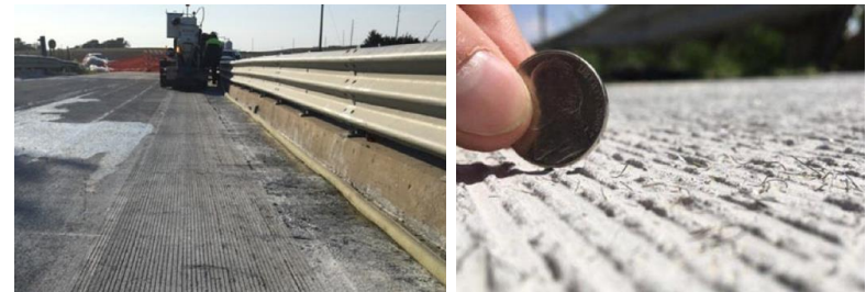
Figure Resource: UHPC overlay on Mud Creek Bridge deck, Iowa, 2017
