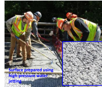
Hydrodemolition (UHPC overlay on Branch Callioon Creek Bridge deck, New York, 2019)
