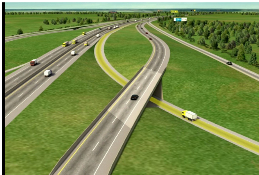
Figure 2-7: Example of a Truck-Car Separated Interchange
