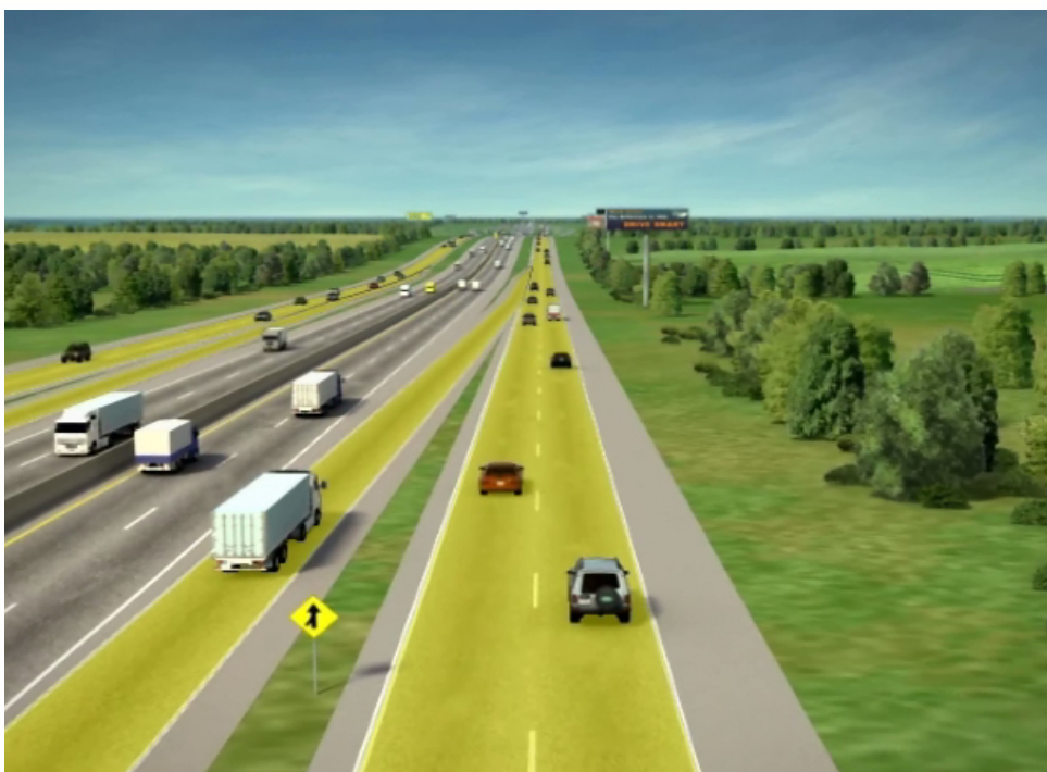
Figure 2-6: Example of a Truck-Only Lane Slip Ramp
