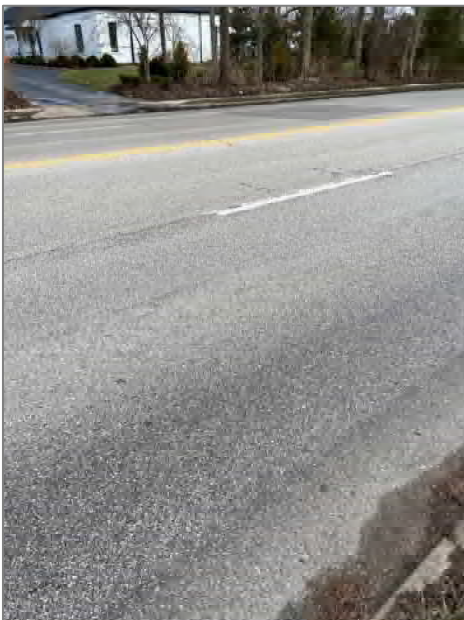
Photo 3: Longitudinal & Transverse Cracking
