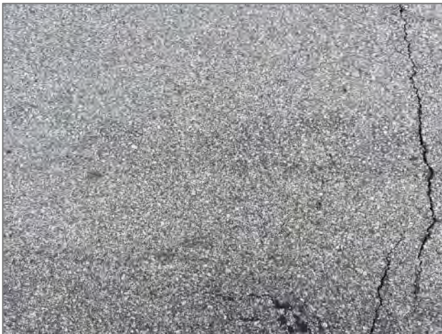
Photo 3: Longitudinal & Transverse Cracking
