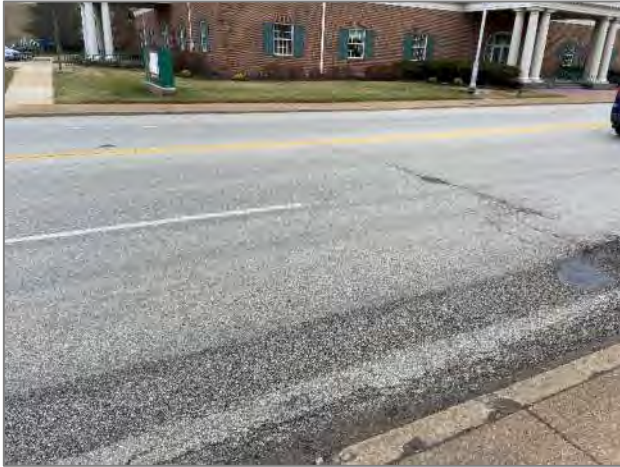
Photo 1: Patching & Polishing
