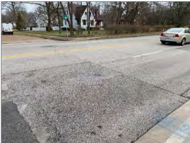
Photo 3: Longitudinal & Transverse Cracking
