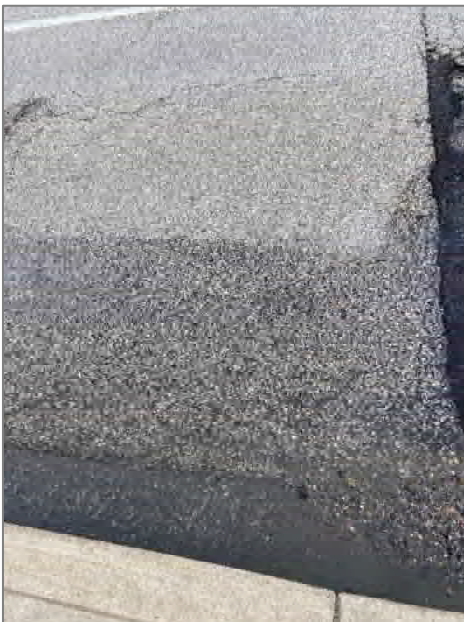
Photo 3: Longitudinal & Transverse Cracking
