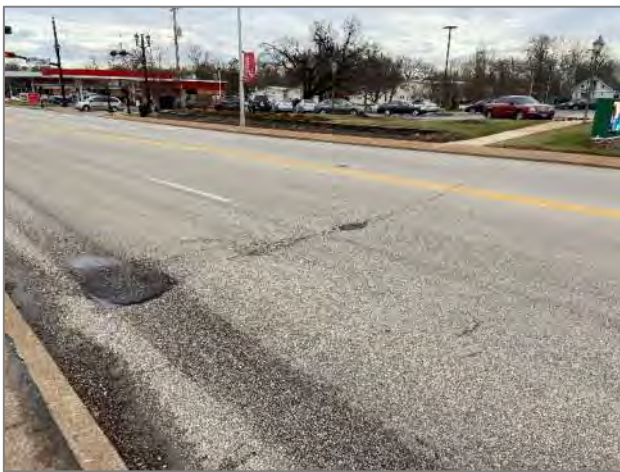
Photo 3: Longitudinal & Transverse Cracking
