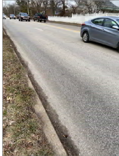
Photo 2: Wheel Path Rutting
