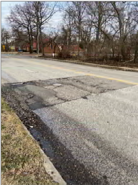
Photo 3: Longitudinal Cracking & Raveling
