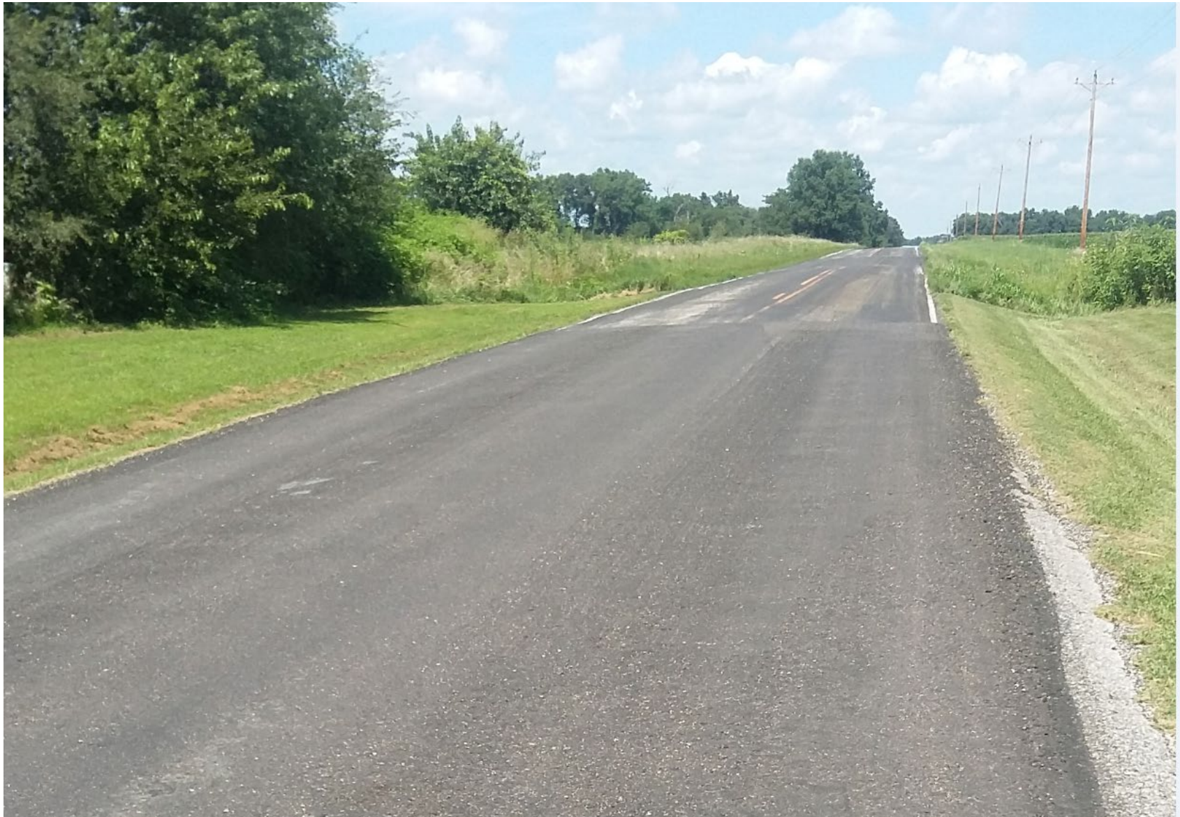
Typical asphalt pavement repair
