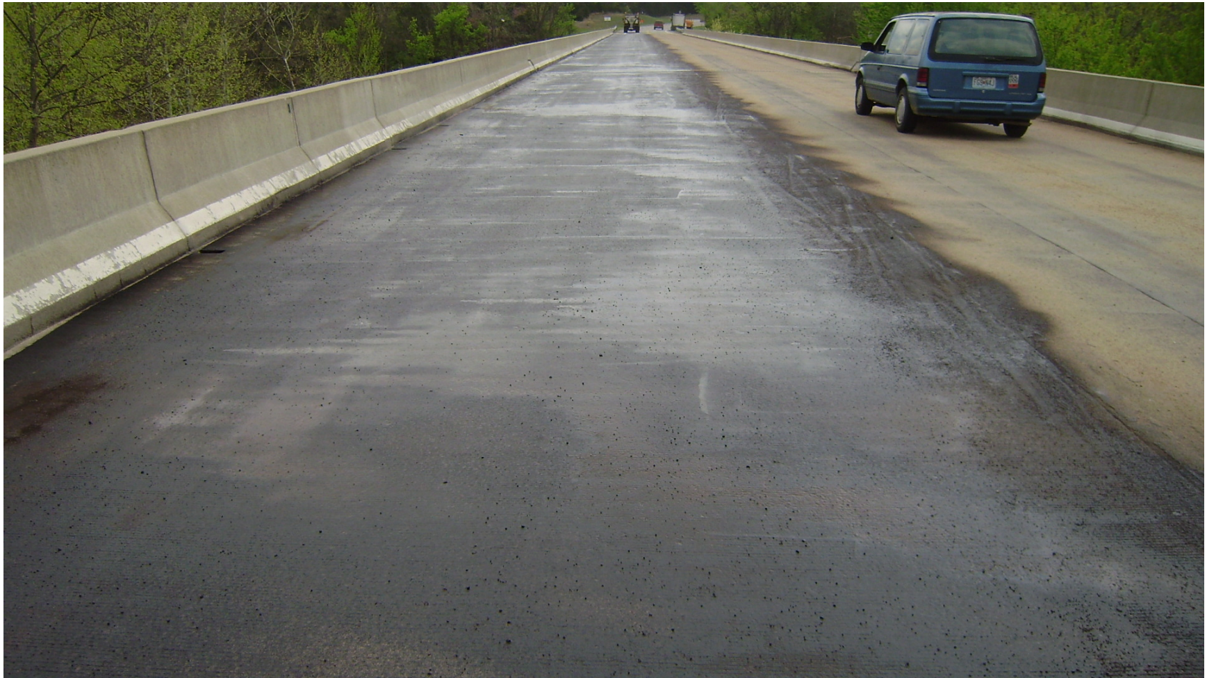
Typical bridge deck seal
